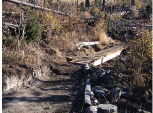
Bridge over a drainage on Yankee Doodle
