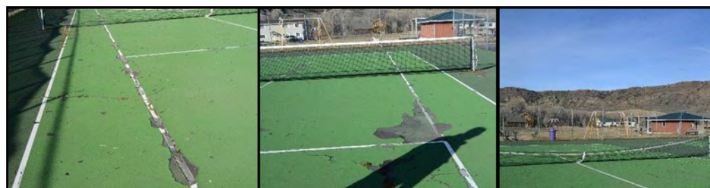
Figure 1: Tennis Court Surfacing
